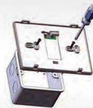
Screw the thermostat back plate on to the back box
